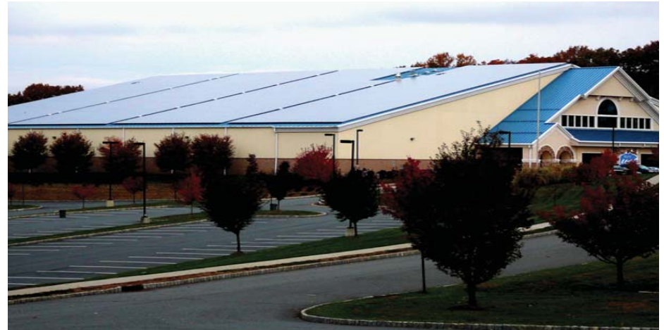
Skating rink in Randolph, NJ. This facility demonstrates how solar panels can be well-integrated into even large commercial buildings. By designing with this in mind, roof penetrations for vents and other rooftop equipment can be concentrated in one area to allow for full coverage of the remaining roof. Photo courtesy of Phil Duran
