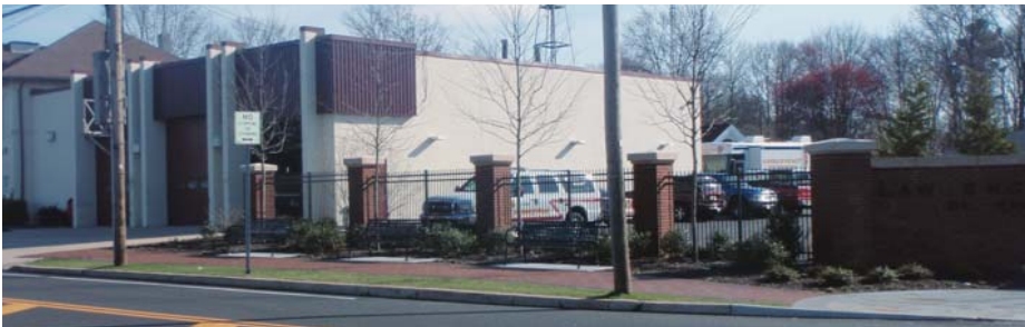
Corner of Route 206 and Marlboro Road, after improvements
