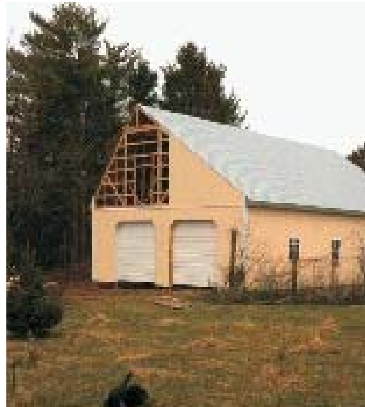
This pole barn in Lawrence Township is being constructed using 95% recycled steel and sustainably grown lumber. The southern roof is larger than the northern one in order to accommodate more solar panels. The roof pitch is set at 8/12 for best solar efficiency. Photo courtesy of Phil Duran
