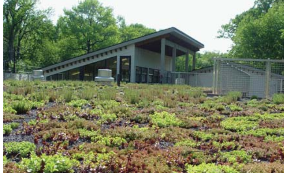
Green roof at the Essex County Environmental Center Photo courtesy of http://www.mgessex.org/cms/index.php?page=green-roof
